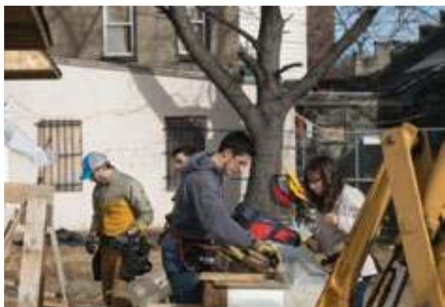
Princeton Seminary students at Habitat for Humanity worksite
